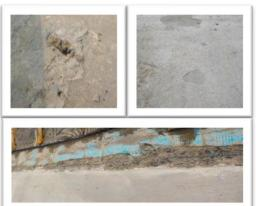
**The solution:** APA were required to provide the application of a proprietary self-adhesive waterproof sheet membrane to the reservoir roof and perimeter upstands. Concrete surfaces were first thoroughly prepared, before a Premseal 100 waterproofing sheet membrane was applied and secured to the entirety of the reservoir roof, upstands and adjacent structure. A
